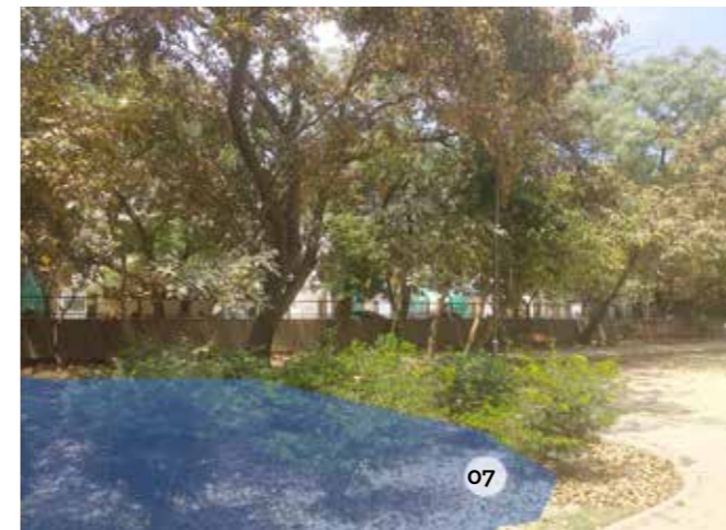
Image 3.15 | Site Image | Rain Water Harvesting Pond
